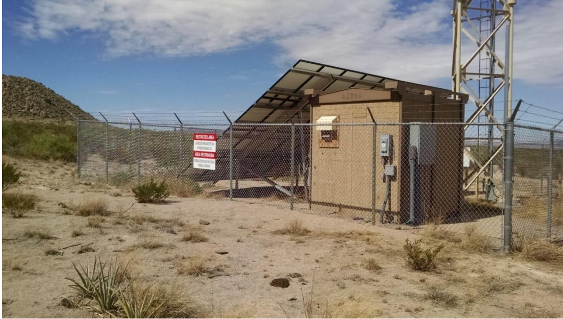
Figure 26. Solar array and power distribution building for the tower.
