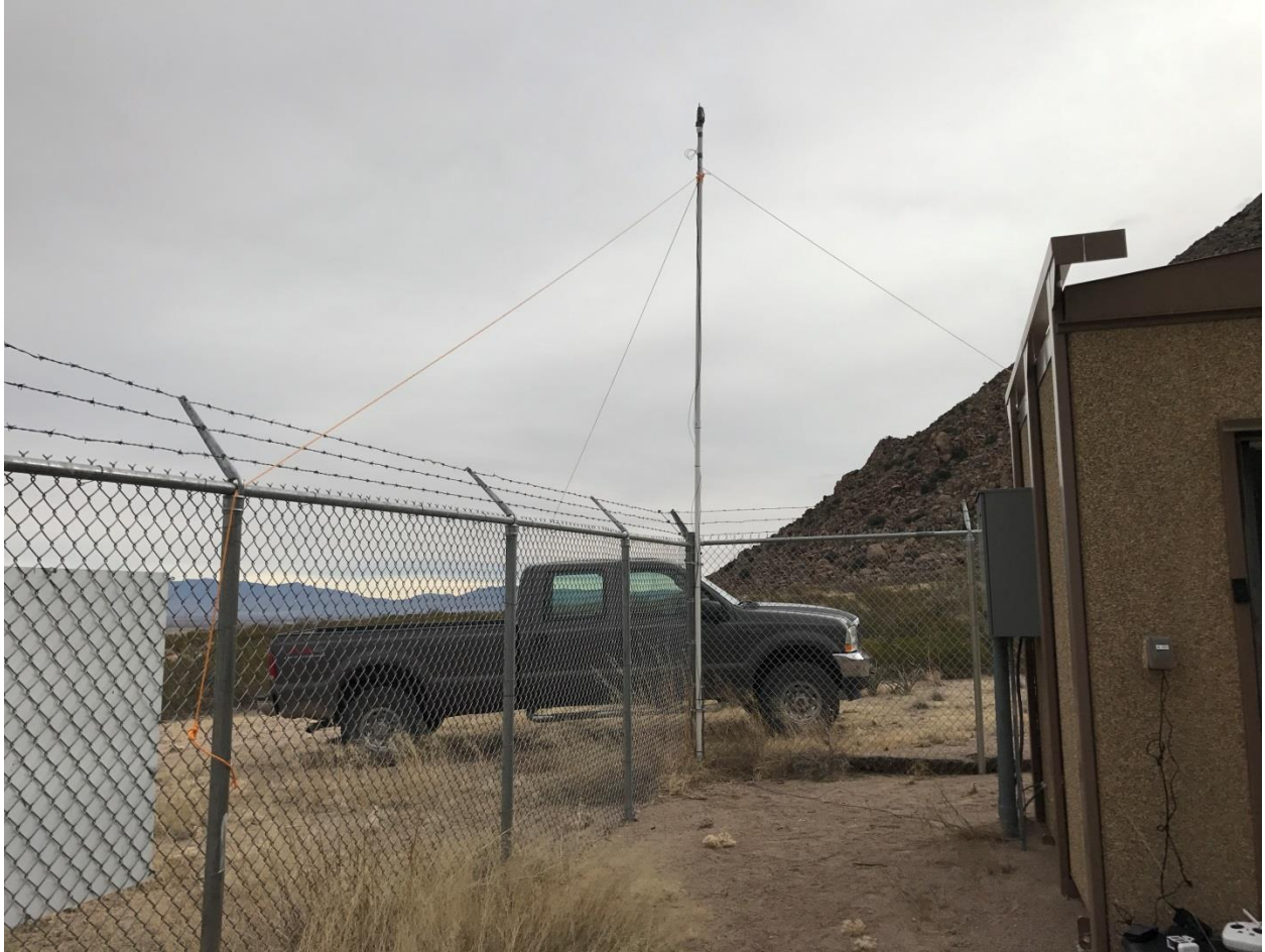
Figure 45. Remote antenna unit at 20 ft AGL, Pole Mast Mount.
