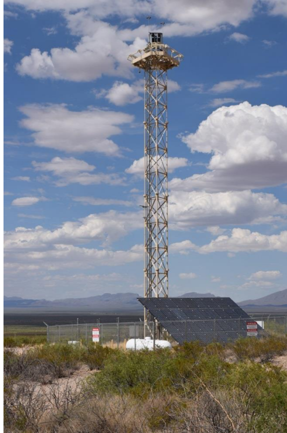
Figure 25. 100 ft research tower—view is approximately to the east.
