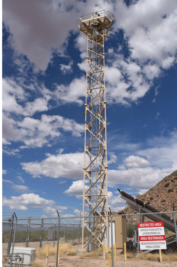
Figure 22. 100 ft tower showing proximity to Summerford Mountain.
