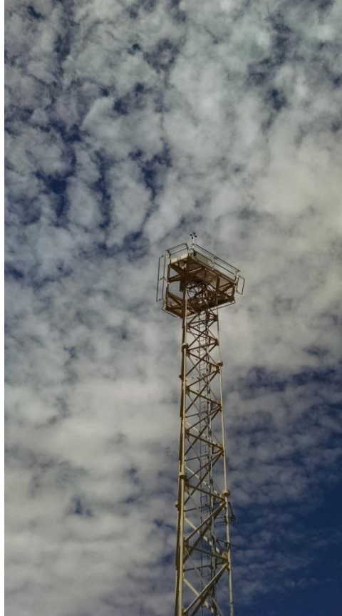
Figure 23. Close-up view of top of the tower.
