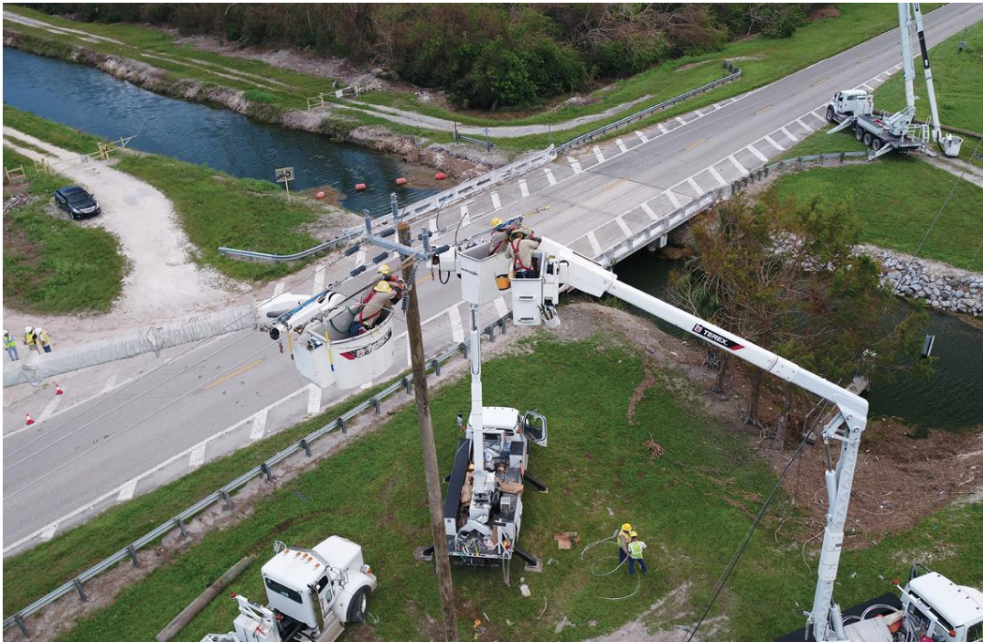
Figure 2. Power restoration work in Florida is documented with UAS following Hurricane Irma, (Knight, 2018).
