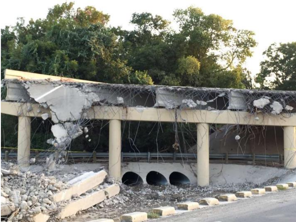
Figure 12. FM 165 Bridge in Wimberley, TX after the flood (Wimberley Strong: 2015 Memorial Day Weekend Flood Wimberley Texas (2016).
