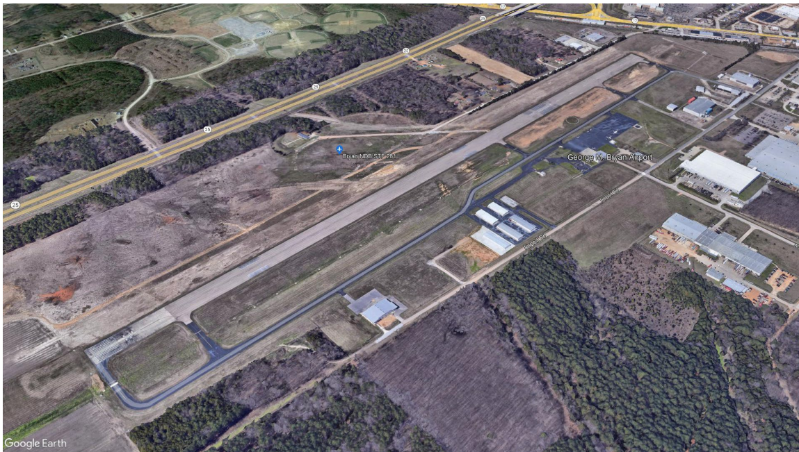
Figure 14. Aerial view of KSTF.
