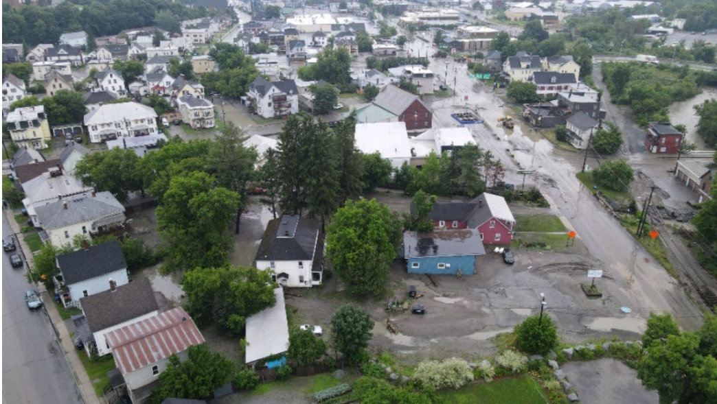
Figure 19. Flood debris and sediment covering Barre City.
