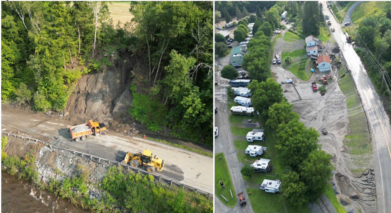
Figure 57. UAS imagery captured along Route 2 in East St. Johnsbury displaying impacts of landslide (left) and washout (right).
