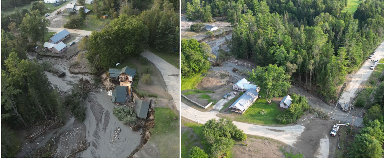
Figure 59. UAS imagery showing significant damage to homes (left) and bridge along Route 114 (right).
