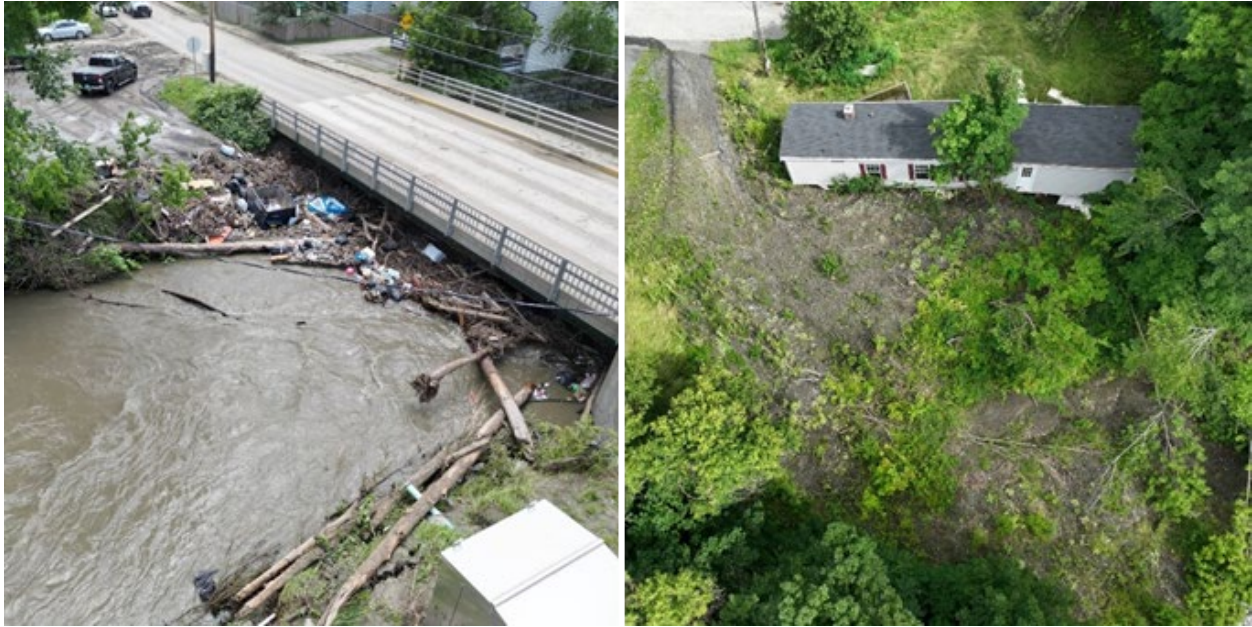
Figure 23. Debris caught in bridge and landslide in residential neighborhood, Barre, VT.
